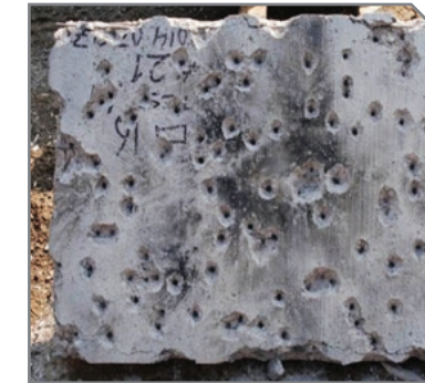
Damage Of RC Slab Under Blast And Fragment Loading
